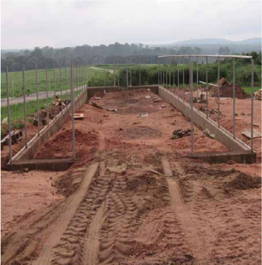
Figure 5. Screen house ground foundation work with the framing.
