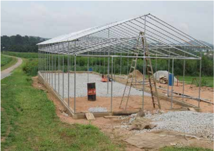
Figure 6. Full establishment of the solid structure for a double ceilings screen house type.
