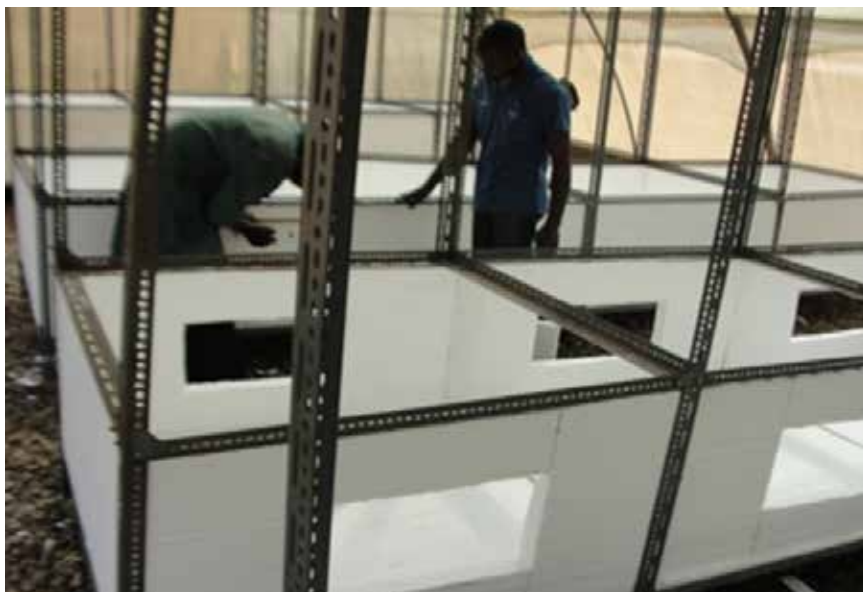
Figure 10B. Construction of the body and windows of aerponics boxes using styrofoam.
