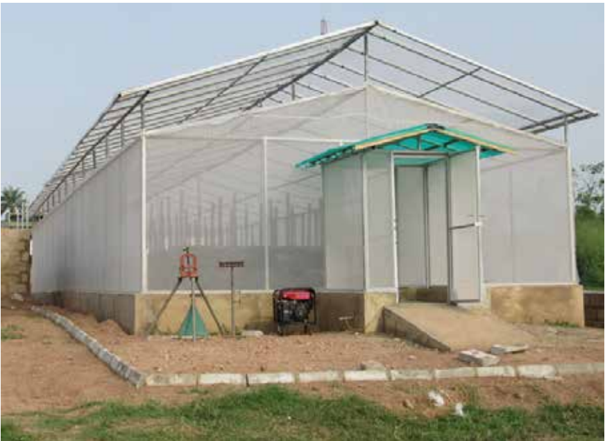
Figure 7. Global view of completed aeronics screen house with double ceilings.
